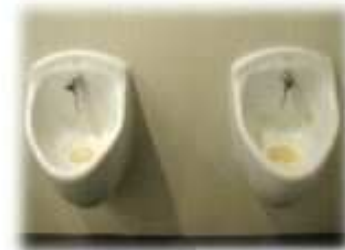
Waterless urinals (with water tap for Muslim users)
